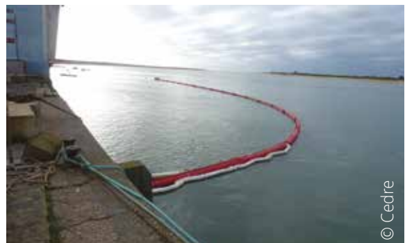
Laying a boom in a chevron arrangement at the port entrance
