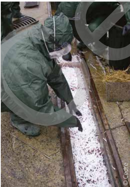
Recovering pollutant using bulk sorbents
