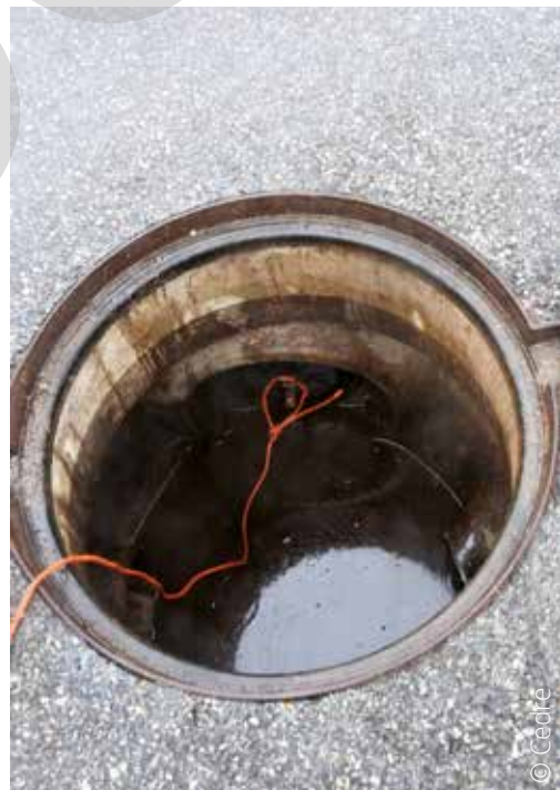
Plugging a manhole
