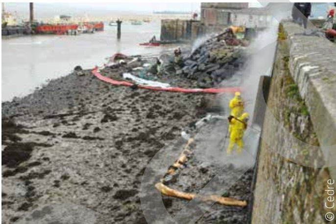
Pressure washing a wall and riprap
