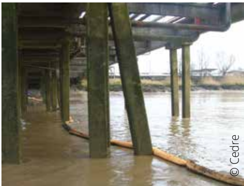
Sorbent boom below a wharf
