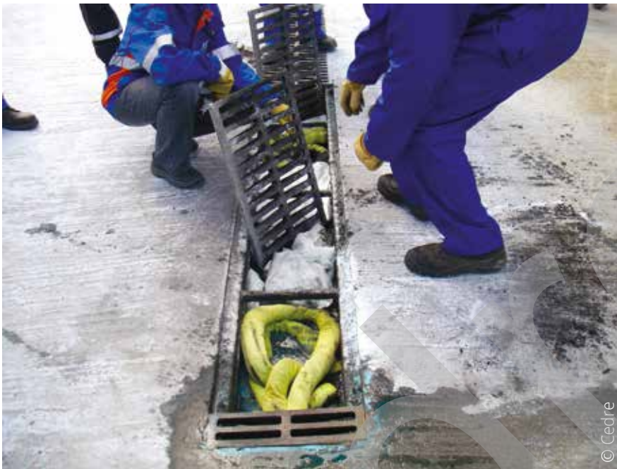
Packing a drain with sorbents
