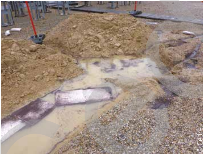
Sorbent pads and peat in a trench to contain an oil spill
