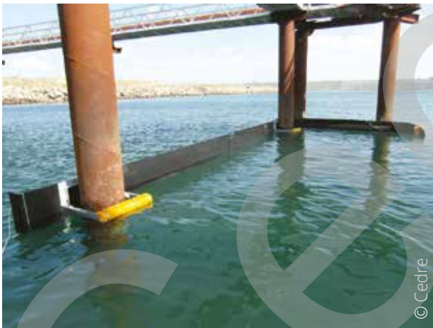
Permanent boom attached to a wharf
