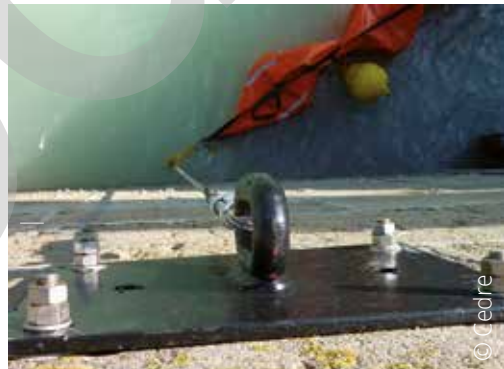
Boom moored to the wire of a tidal compensator
