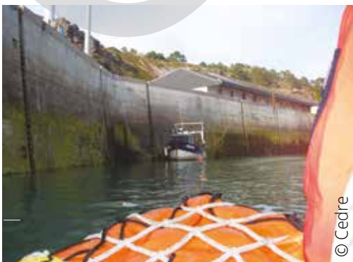
Boat-based survey along a quay wall
