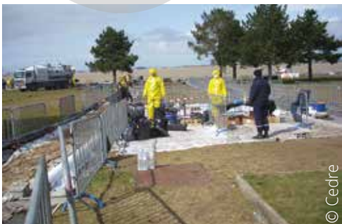
Walkway and logistics area
