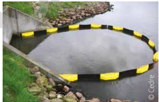
A permanent boom installed at an outfall
