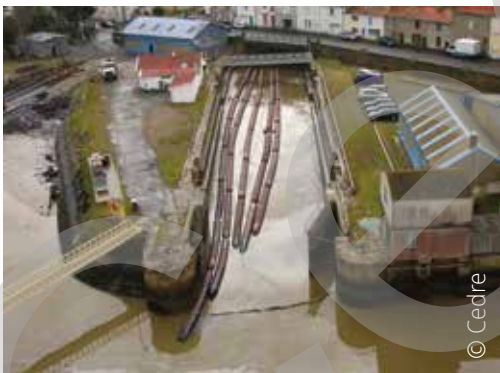
Oiled harbour basin and pipes
