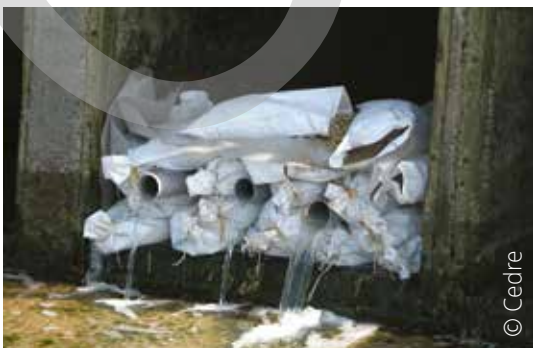
Containment and water level management with a dam made of bags of rubble
