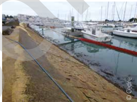
Oiled quay and containment using booms
