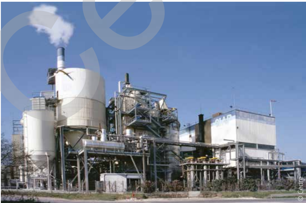
Hazardous waste treatment plant
