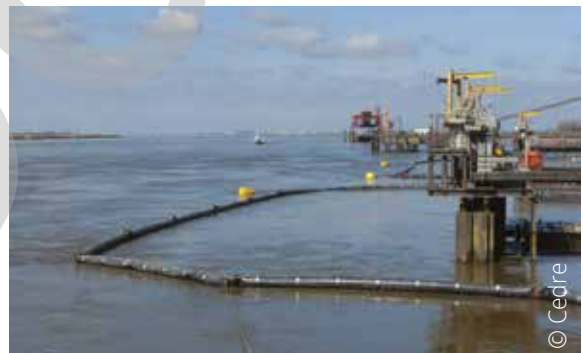
Laying a boom as a preventive measure to protect quays
