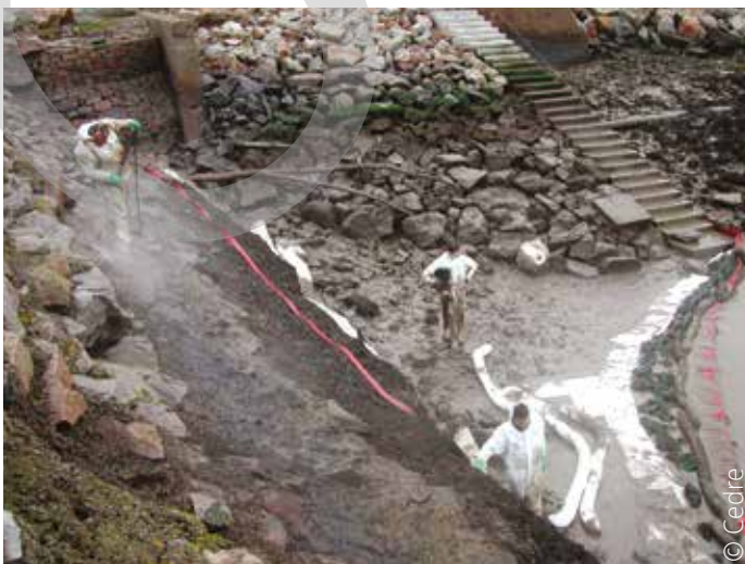
Recovering washing effluents using sorbent pads, pompoms and booms
